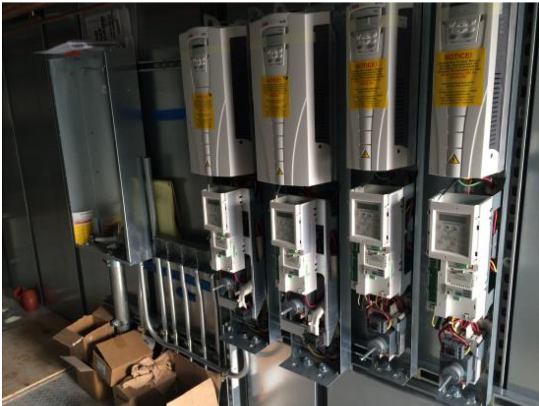
VFD's are mounted and piping is underway in AHU 4. (Yellowstone Electric)
