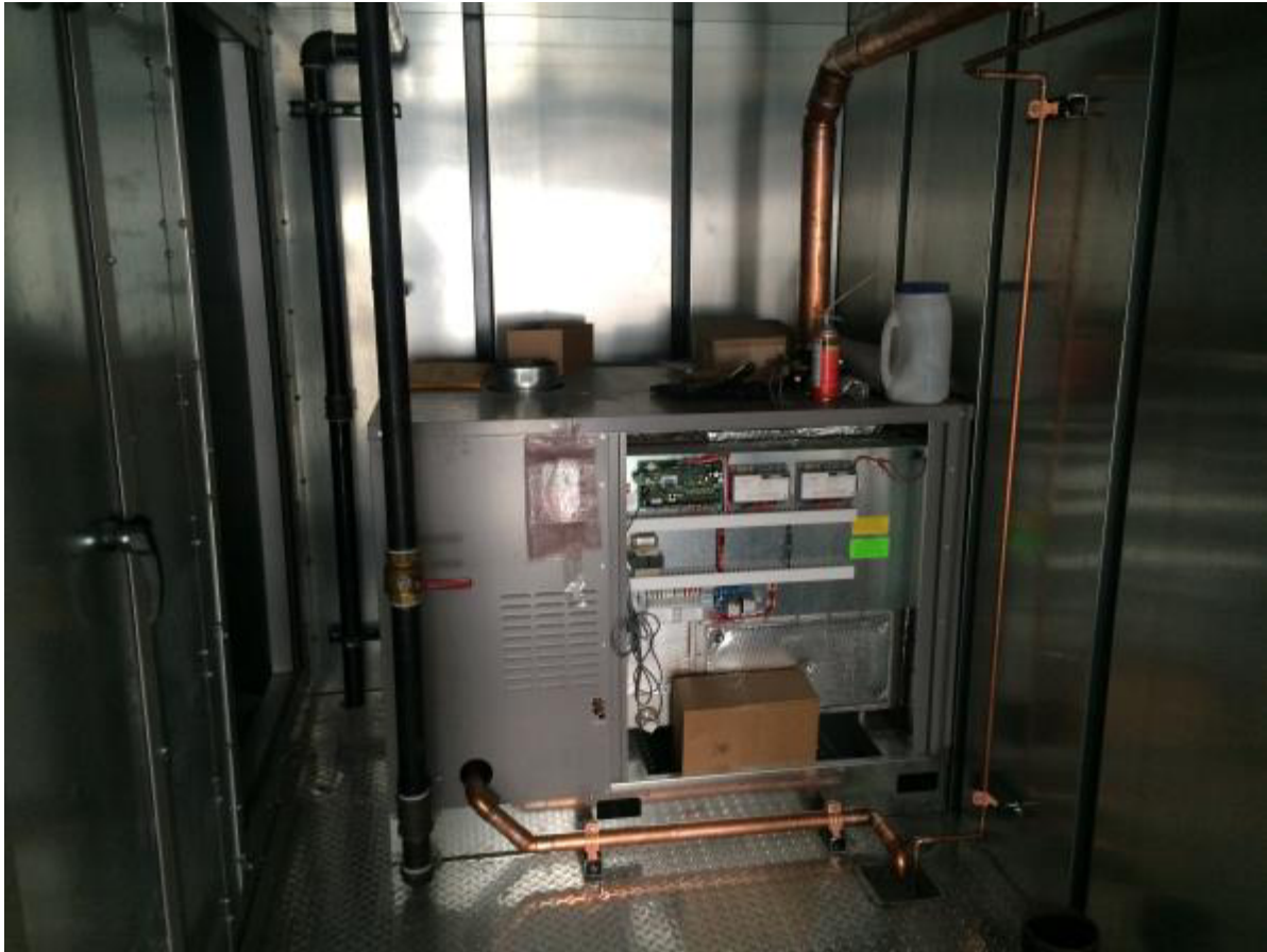
Piping for the Humidifier in AHU 4 is underway. (Basin Mechanical)
