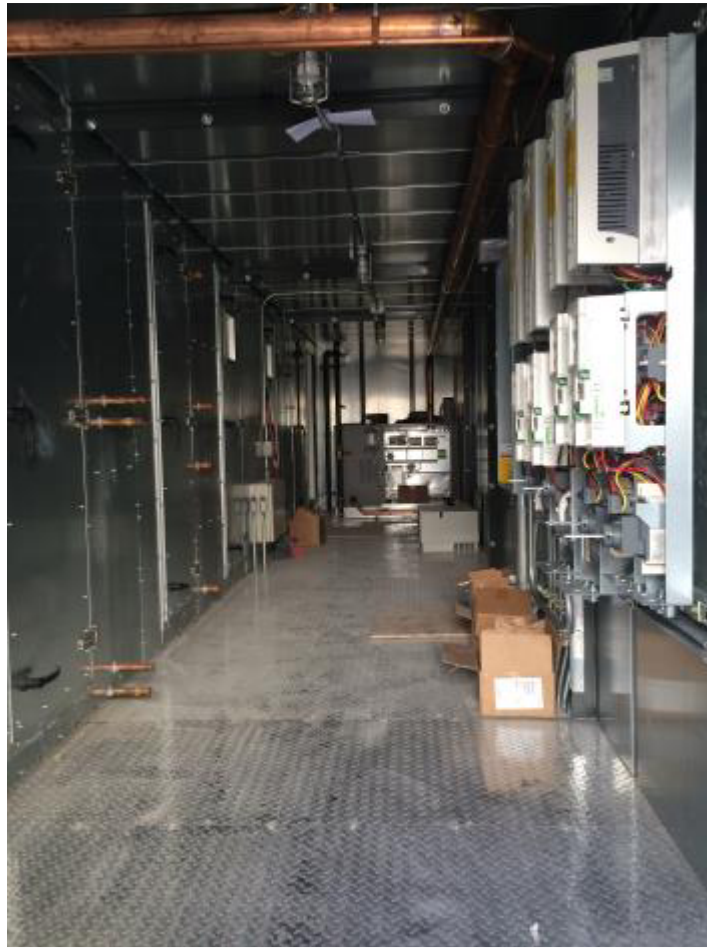
AHU 4 rough in is underway. (Basin Mechanical/Yellowstone Electric)
