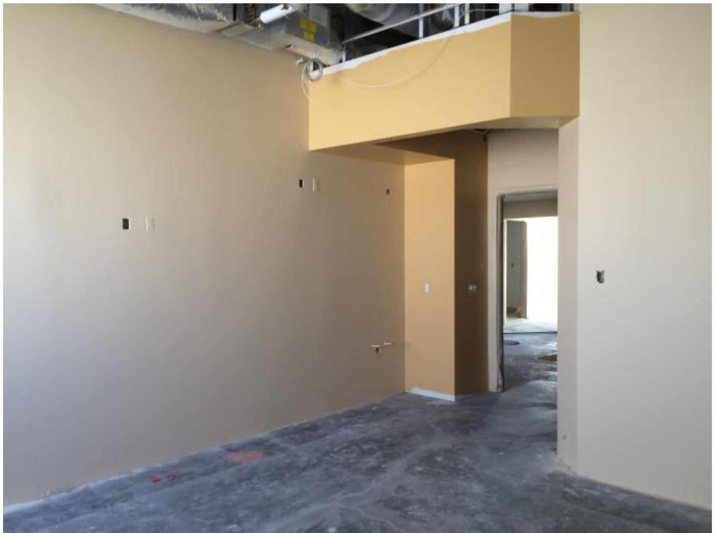
1 st coat of paint in patient room. (Excel Painting)
