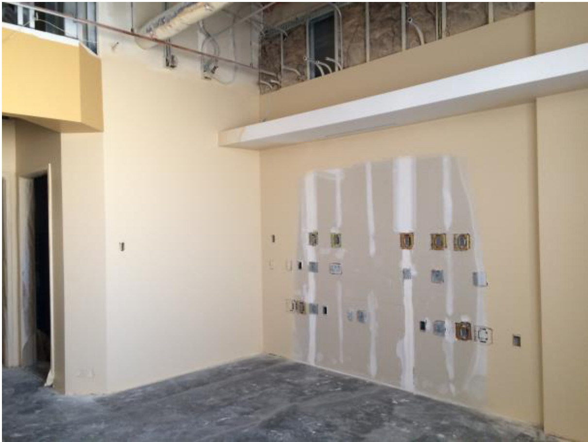
1 st coat of paint in patient room head wall. (Excel Painting)
