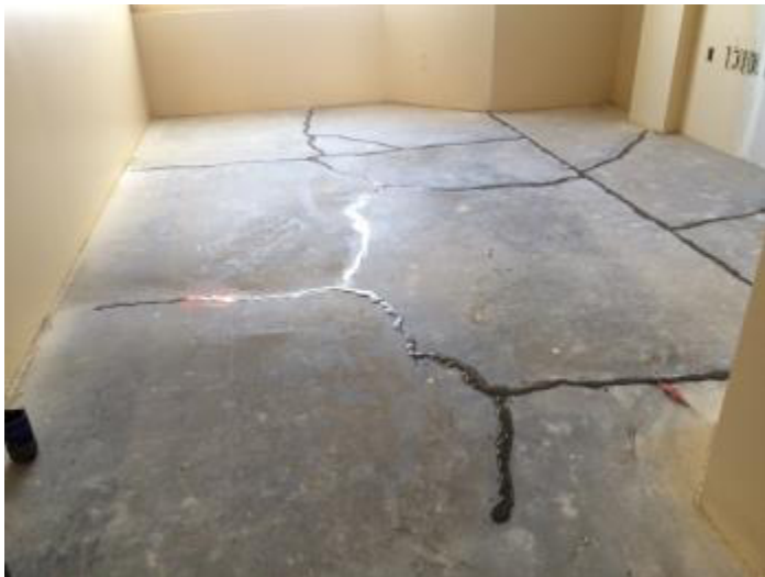
Crack isolation and floor prep is underway. (All Commercial Floors)
