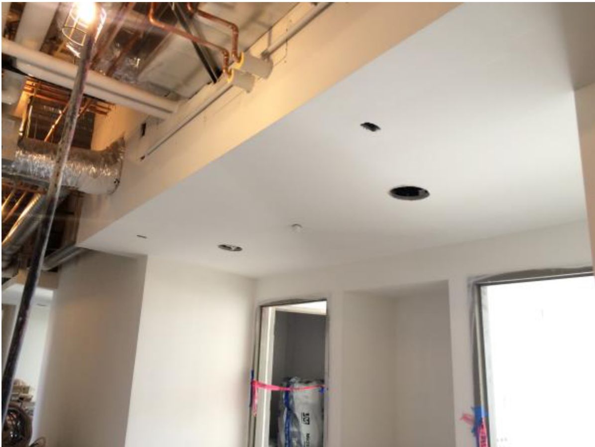
Soffits on the North side are complete. (Empire Lath and Plaster)
