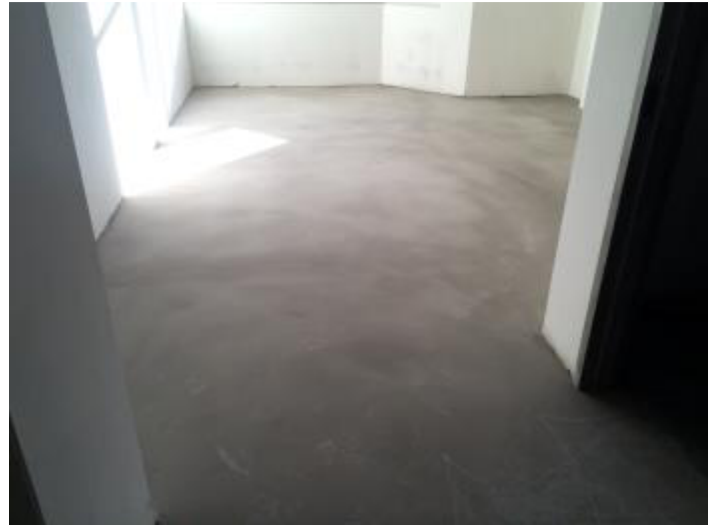
Crack isolation and floor prep is underway. (All Commercial Floors)
