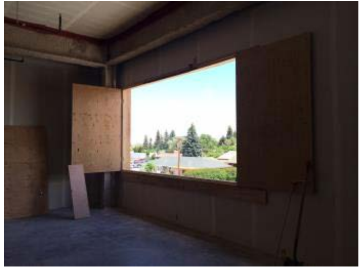
Window has been removed and opening is protected with doors. (Cowan Construction)
