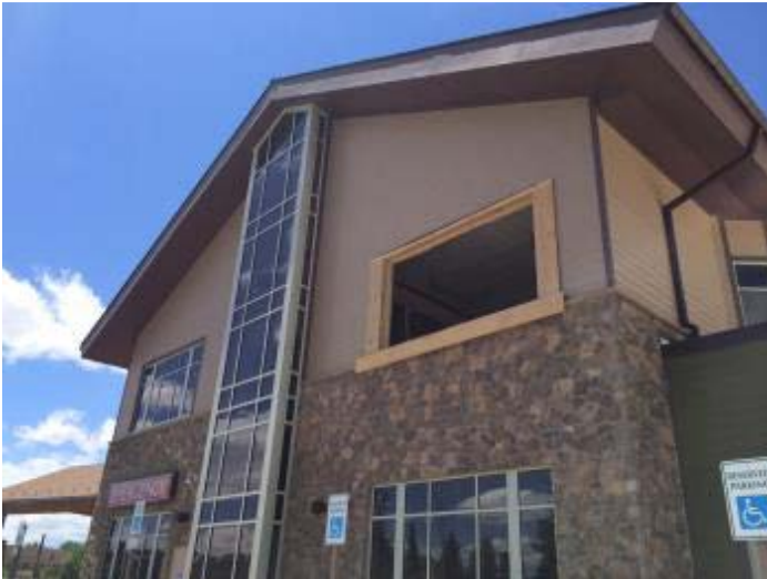
Window has been removed and opening is protected with doors. (Cowan Construction)
