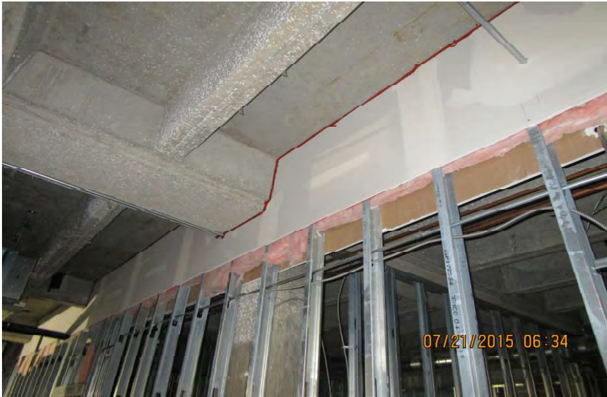
Cedar Mountain Top-out and Fireproofing
