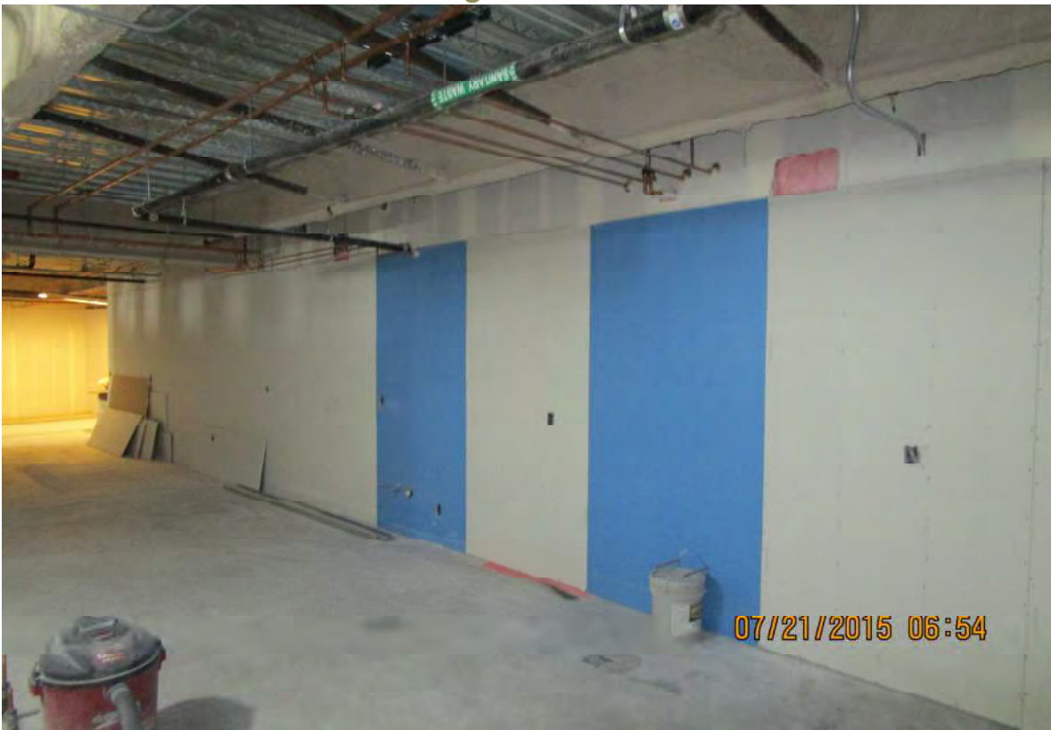
Dietary Area A Dry Wall
